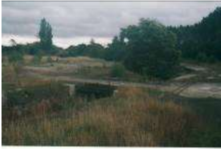
Bridge at West Beck
