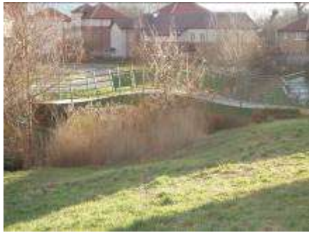
West Beck bridge
