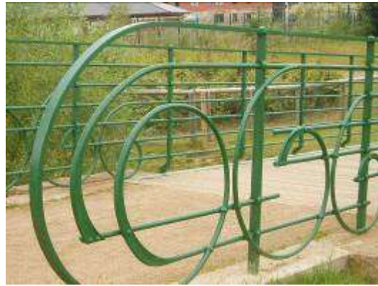
Figure 15: Main bridge (Village Gate)
