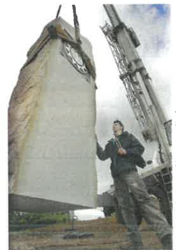
David Paton inspects the first sculpture being installed
